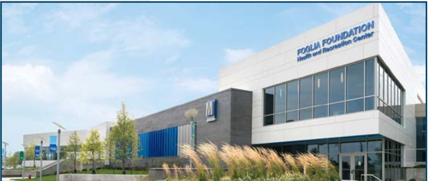
Foglia Foundation Health and Recreation Center at Harper College
